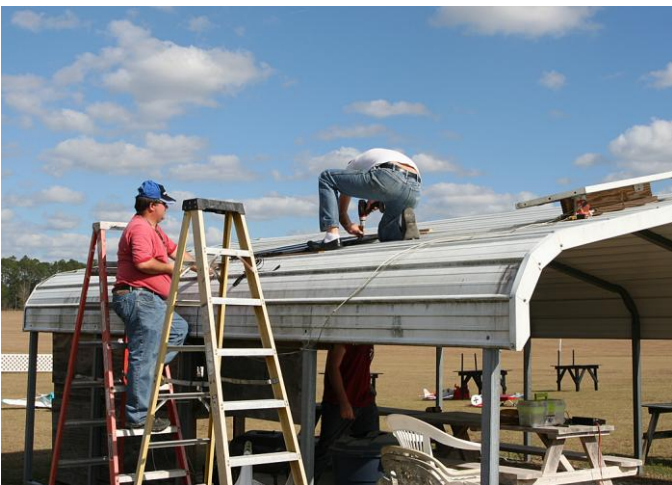
Curtis and Norman installing the new solar panels
